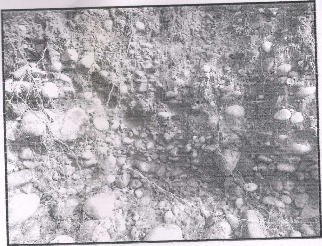
1.11 Image showing exposed rock mass along the road cutting.
